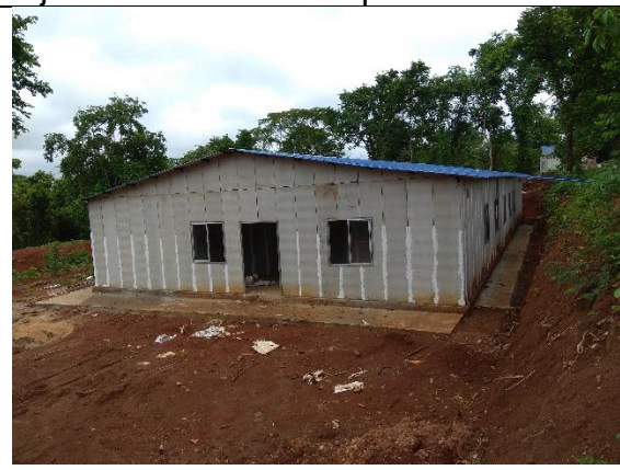
Hospital / First Aid Centre
