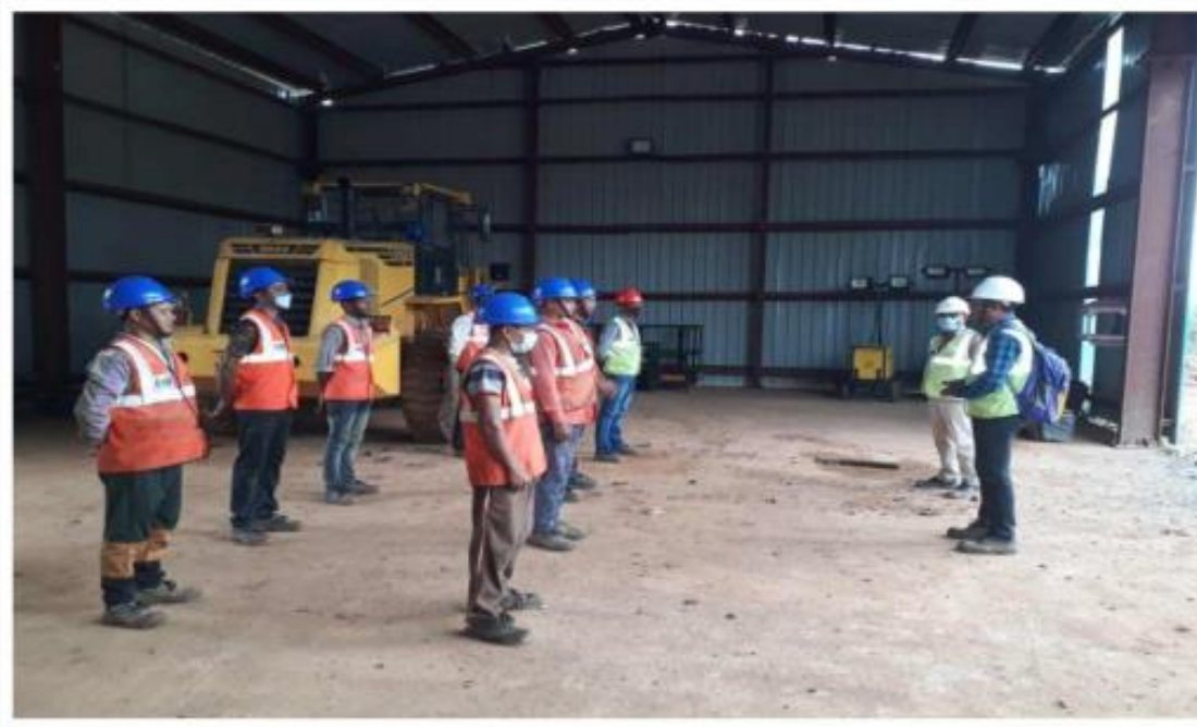
Fig- 60,61,62 &63 : EHS briefing before start of work every day before start of work.
