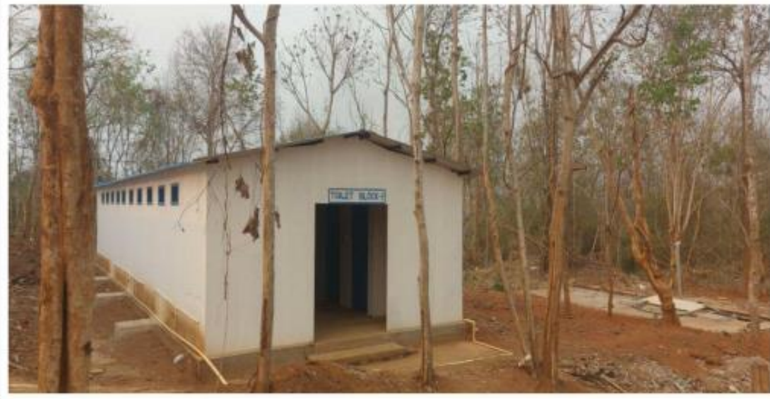
Fig- 57 &58: Toilet block for Lohit & Manas camp completed.
