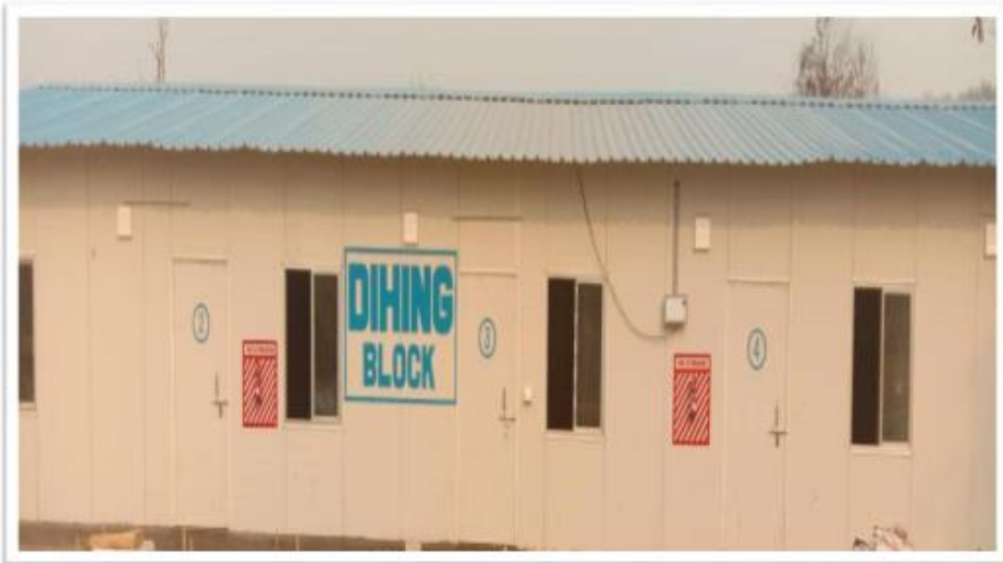
Fig-44: Fire Extinguisher kept in Dihing Block (Employer/PMC Accommodation).
