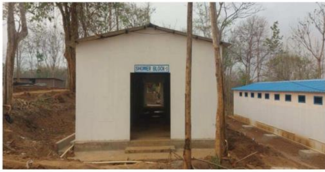
Fig- 56: Shower Block for Lohit & Manas camp completed.
