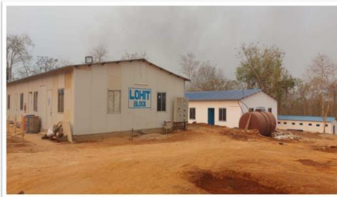
Fig- 54: Lohit Block (Worker camp) Completed.
