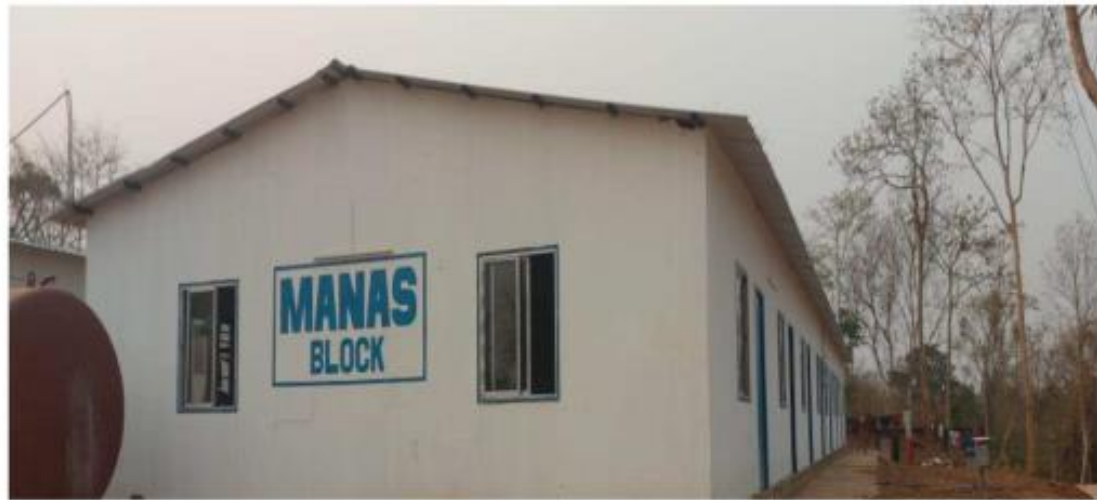
Fig- 55: Manas Block (Worker Camp) Completed.
