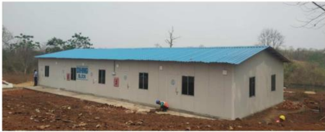
Fig-59: Employer /PMC Accommodation ready for possession (Dihing Block).
